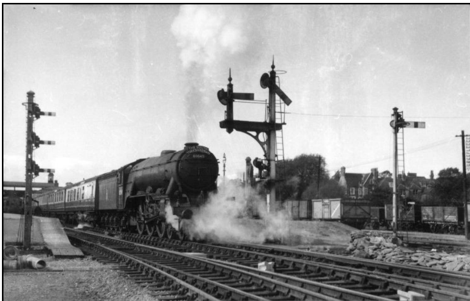
Class A3 4-6-2 no. 60049 'Galtee More' starts away from Aylesbury with the up 'South Yorkshireman'.
