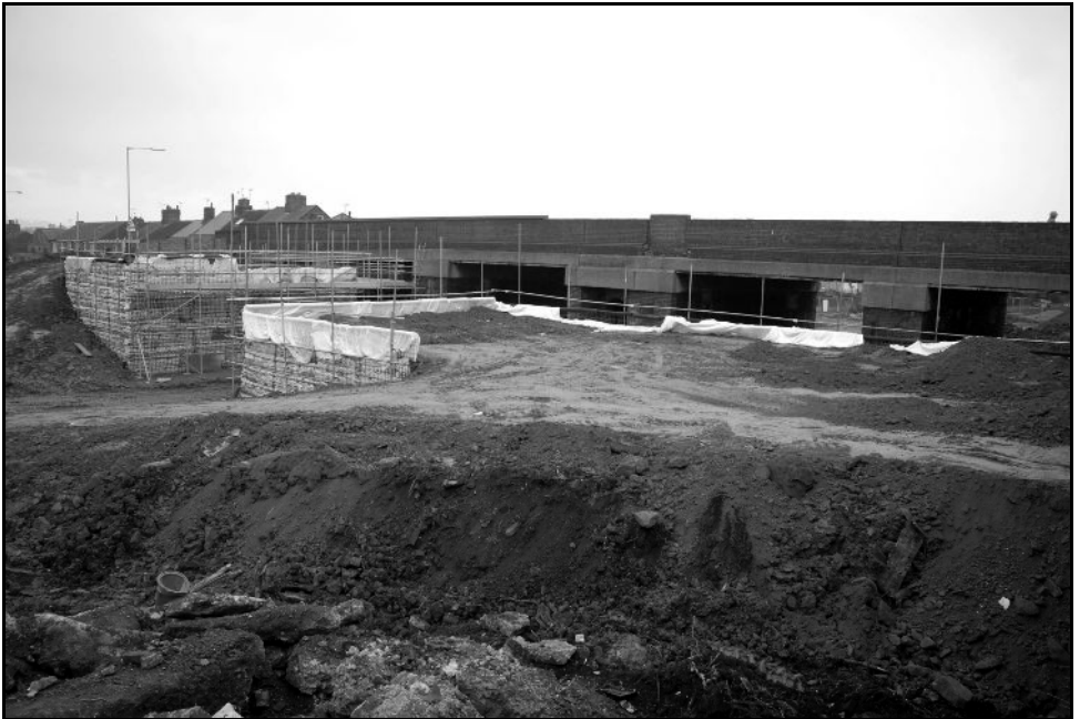
View from the cattle dock showing the new bridge taking shape.
