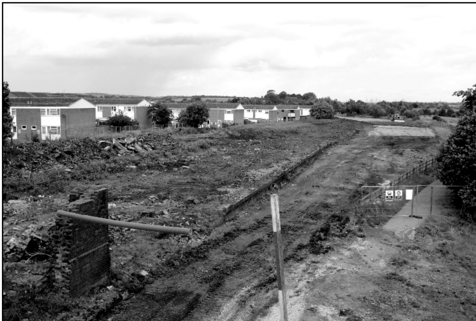
The view of Staveley station site looking north from Lowgates bridge on 21 June 2007. The brick footbridge support and the edging stones on platform 2 can still be identified. The blocked off Beighton-Staveley Trail is on the right.
